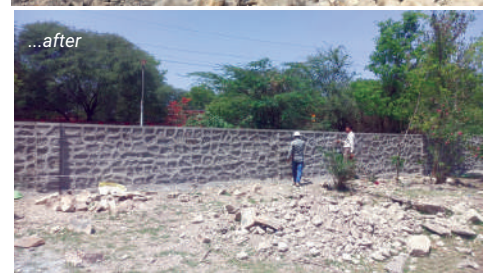
Repair of Boundary Wall
